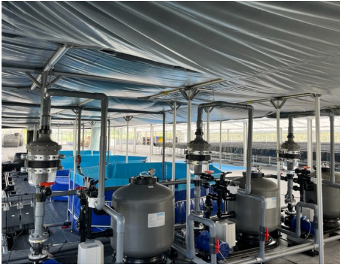
Aquabiome ASM600, MultiCyclone 16 and UV Solclear installed at Aquaponi's sturgeon and tilapia farm
