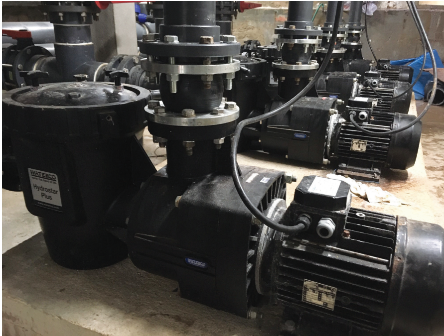
Waterco's Hydrostar Plus 7.5kW pumps upgraded with silicone carbide seals are ideal for sea water installations.
