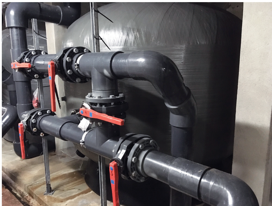
CIMAI chose Waterco’s reinforced fibreglass filters and injection moulded thermoplastic pumps to replace the antiquated equipment.
