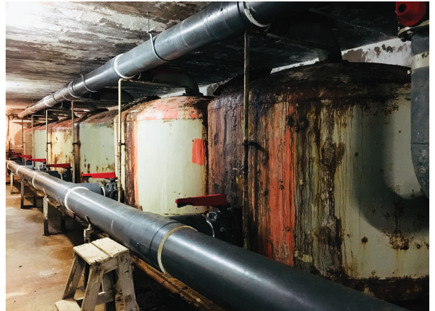
Ongoing contact with seawater caused the pool's filters, pumps and metallic components to rust.
