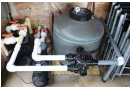
Micron side mount fibreglass filter filled with Waterco Glass Pearl filter media and a Lacronite pump.
