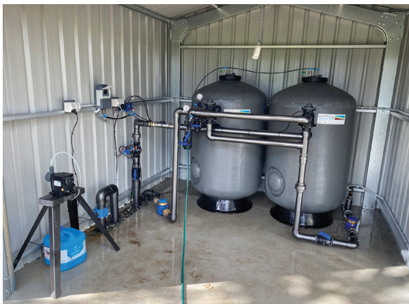
Students and teachers at Joondalup Primary School now have an effective bore water treatment system by Waterco and Earth & Water.
