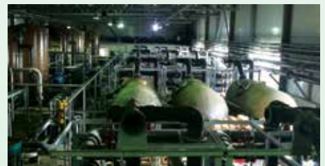
Waterco was awarded the contract to provide 12 Micron MD10,000 horizontal filters. These 7-bar rated filters are made using the latest in fibreglass winding technology and use the highest grade of non-corrosive materials.
