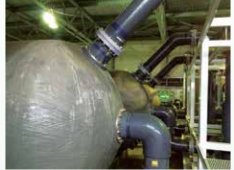
Waterco's filters are designed with no metal to water contact and are suitable for a long service life due to the high pressure rating.
