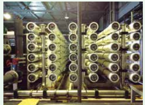
10,000 m 3 /d seawater reverse-osmosis (SWRO) desalination plant to support the drinking and process needs of local residents and the new Far Eastern Federal University.
