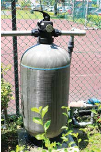
When you have children facing serious health challenges, clean, healthy water is essential to their recovery. A high quality filtration – Micron Deep Bed Sand Filter was recommended by Waterco as a solution.
