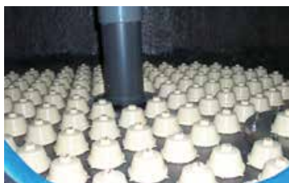
Nozzle Plate under drain system
