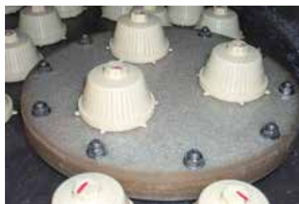
Internal Nozzle Plate Service Hatch
