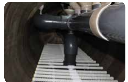
Internal plumbing & laterals
