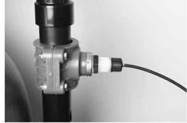
Figure 6.12 Connecting acid feed line to the injector
